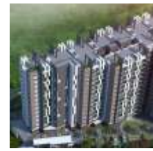
DSR RR Avenue Mumbai Hwy, Bengaluru
