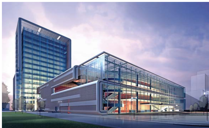
Commercial Tower with Retail and Office Spaces on Radial Road # 4 @ Narsingi
