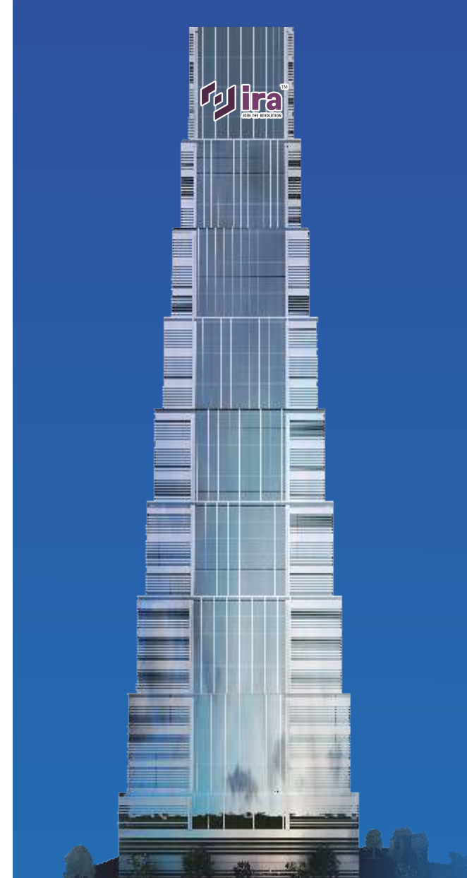
GATEWAY TOWERS, PUPPALAGUDA
